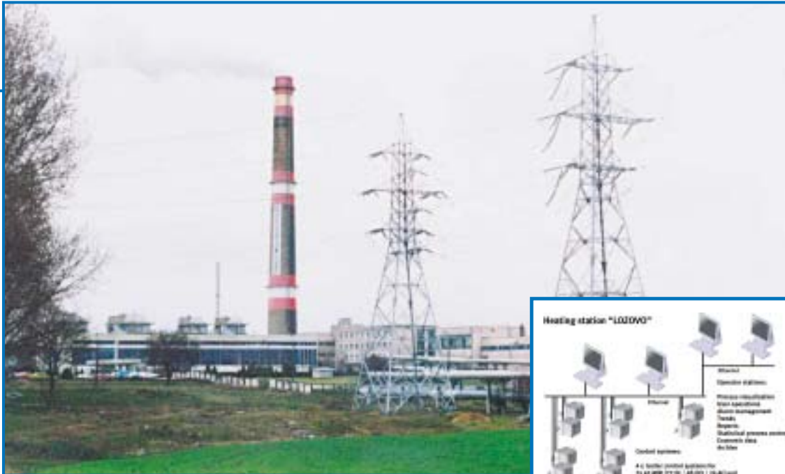
The heating plant Burgas
