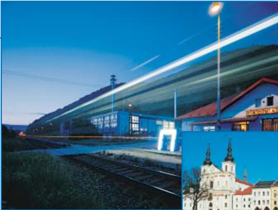
Night view of the district heating plant Radvan, Slovak Republic
