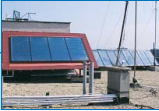
Thermal solar collectors for hot water preparation on the roof of a house
