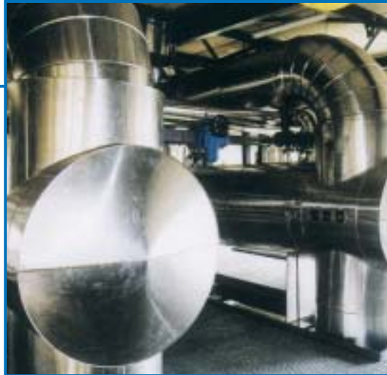
Steam boilers in Ravne, Slovenia
